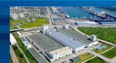
Donghae Plant Submarine Cable Industrial Specialty Cable
